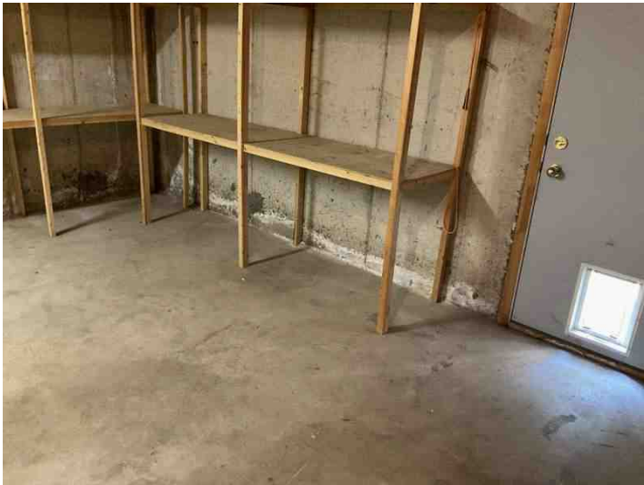
Unfinished Basement Area
