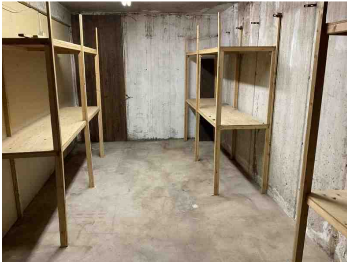
Unfinished Basement Area
